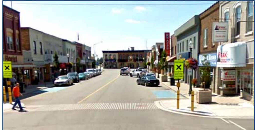
Left: Painted zebra stripes or cross-hatching indicate the crossing area. Right: Curb extensions decrease the pedestrian crossing time and increase their visibility. (Listowel, Ontario. Both Photos Courtesy of Google Street View 2012. Accessed August 29, 2012 through maps.google.ca)
