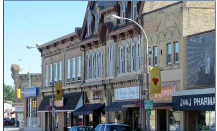
Second-storey windows are aligned, and cornice lines distinguish the storefronts from the upper storeys. (Clinton)
