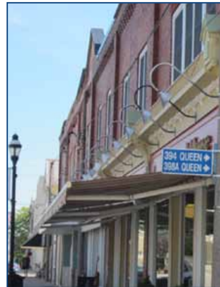
Awnings and lighting create a comfortable pedestrian environment. (Blyth)
