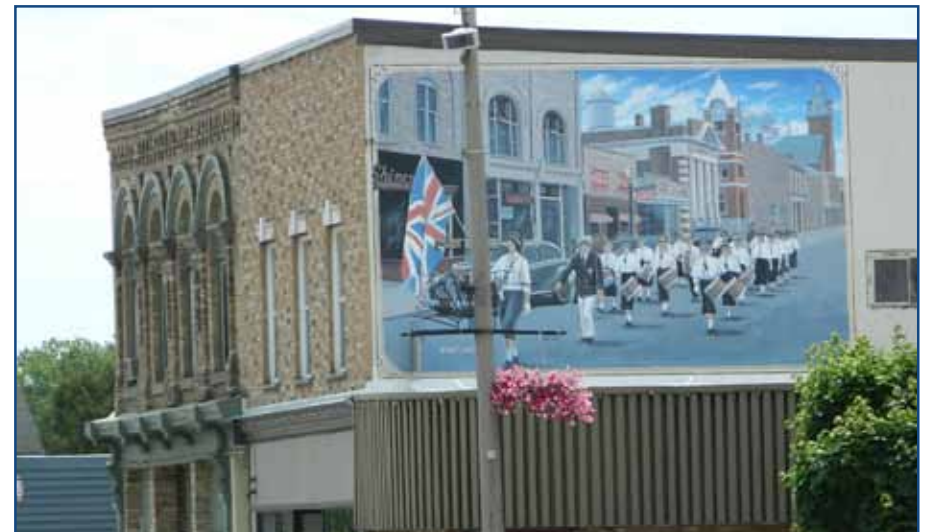
Top: Paintings decorate filled-in windows on a side wall. (Clinton) Bottom: The mural on the side of the second storey of this building enhances an otherwise blank wall. (Seaforth)
